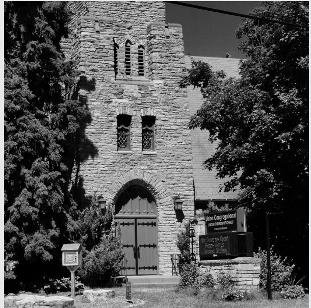
Below, current Union Congregational Church, built, 1941.
