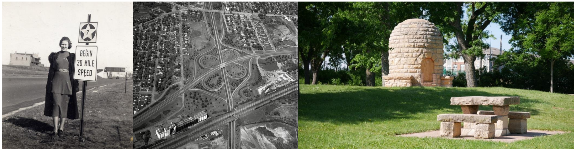
Marie Hartmann, (left), founder of the St. Louis Park Historical Society, stands along Highway 7 shortly after it opens in the mid-1930s. The Highway 7-Highway 100 cloverleaf was a traffic engineering marvel, shown in this aerial photo with the Commodore Elevator lower left and Minnetonka Blvd, top. Highway 100 was landscaped with lilacs and became known as Lilac Way through the western suburbs, and roadside parks, such as the restored Lilac Park west of Nordic Ware, provided picnic venues for the accelerating automobile society, post-WWII.
